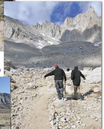
Citizen-stewards from Volunteer Vacations rehab campsites at Trail Camp on the Mt. Whitney trail.
